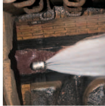
High pressure flushing nozzle cleaning a sewer
