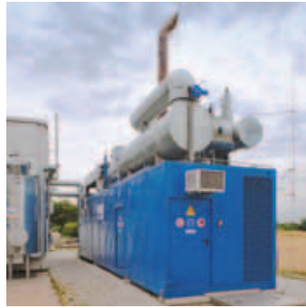
Combined heat and power station in a container
