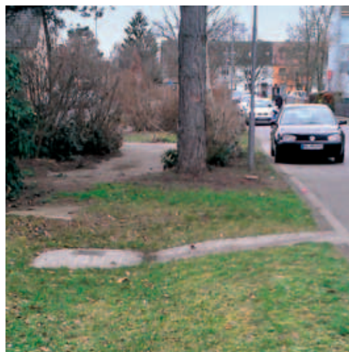
Percolation trough in the public roadside environment
