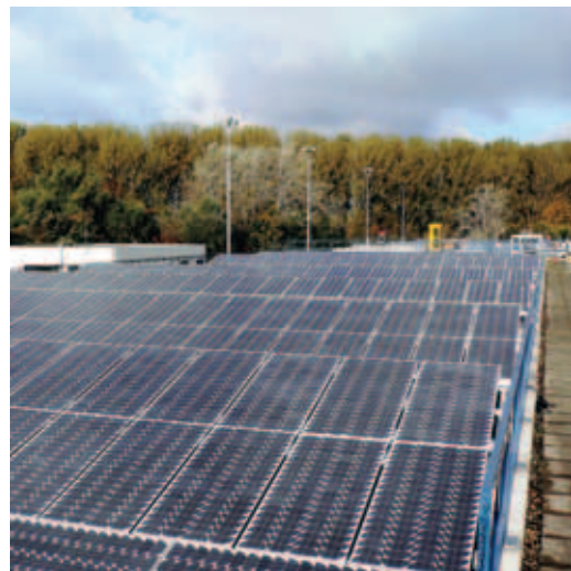
Photovoltaic installation on the filtration section
