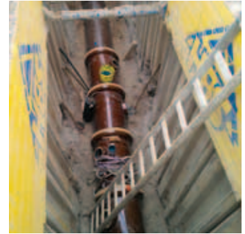
Sewer being laid in a pit
