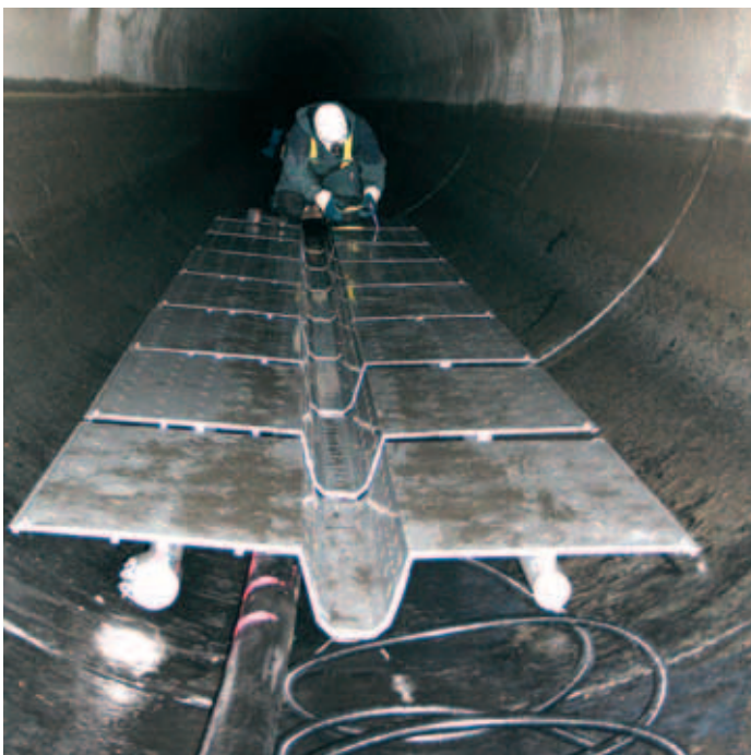
Heat exchanger in the sewer
