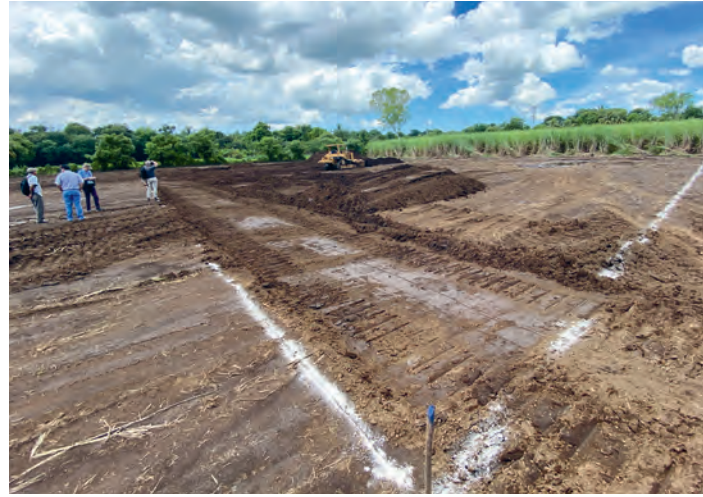
Preparatory work for the construction of the infiltration basin in El Viejo
