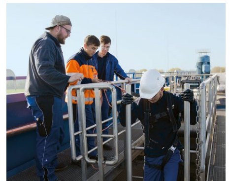
Trainee carrying out checks on the digestion tower roof
