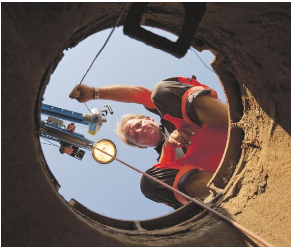
Preparing to survey the sewer with a camera
