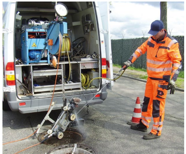
Cleaning the sewer camera
