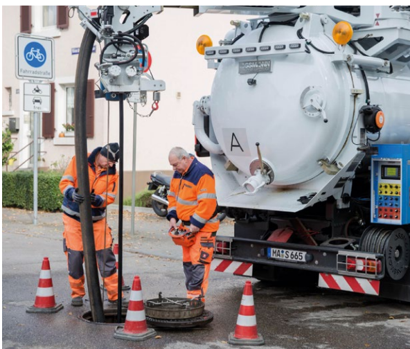
Cleaning team preparing for work at the open sewer maintenance shaft
