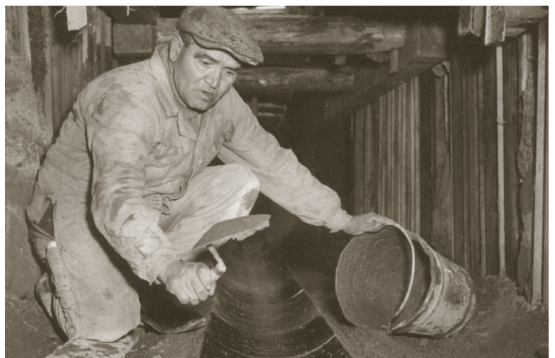
Mason working on the sewer bed lining in 1951
