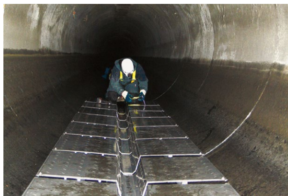
Heat exchanger in the inlet sewer to the Ochsenperch pumping station
