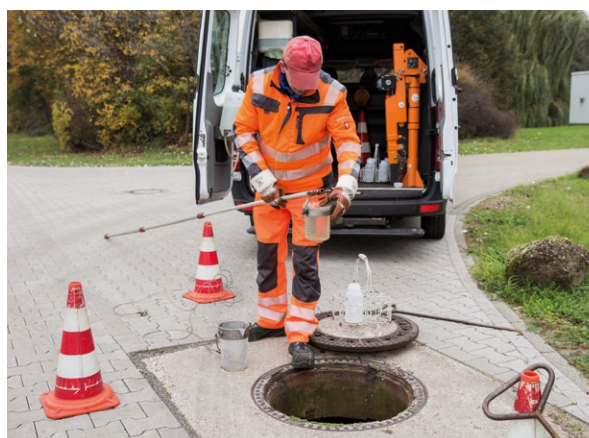
Taking samples at the manhole of an indirect discharger
