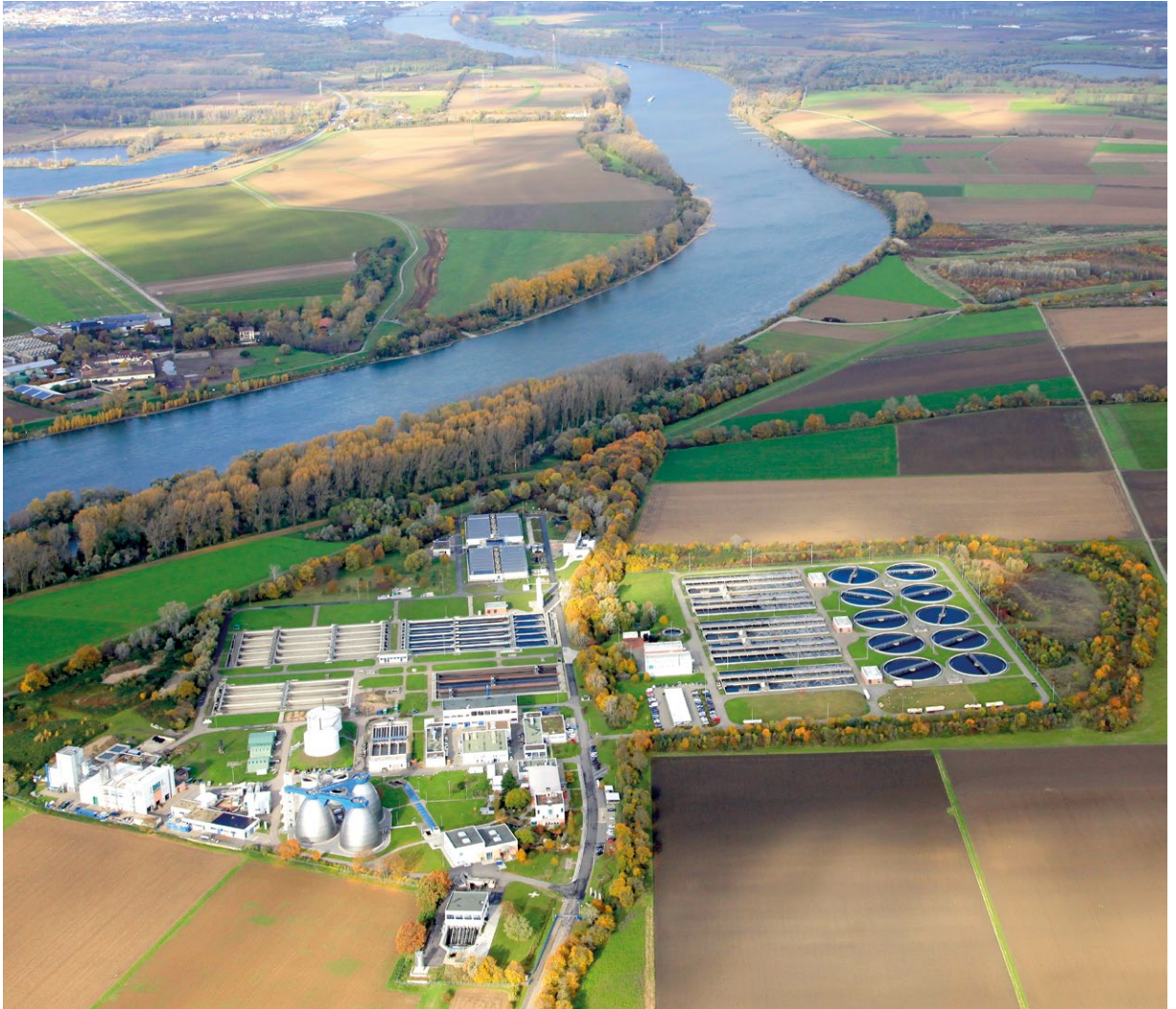
Aerial picture of the treatment plant in 2019
