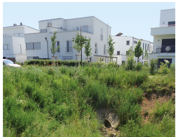
Rainwater infiltration ditch at the Am Hochwald construction site
