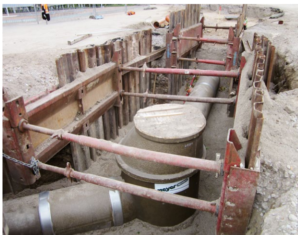
Round shaft with connected sewers in the open trench
