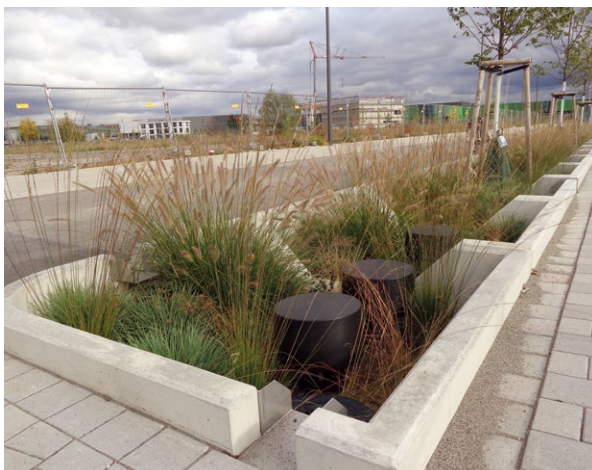
Rainwater infiltration in a deep bed on the Taylor Barracks site
