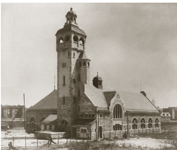
The Ochsenperch pumping station in 1904
