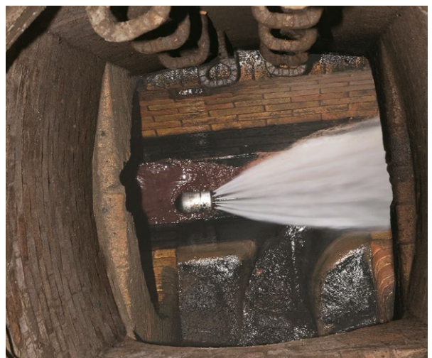
Sewer cleaning with high pressure jets
