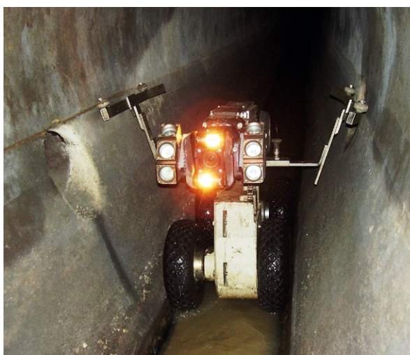
Remote control sewer camera in use
