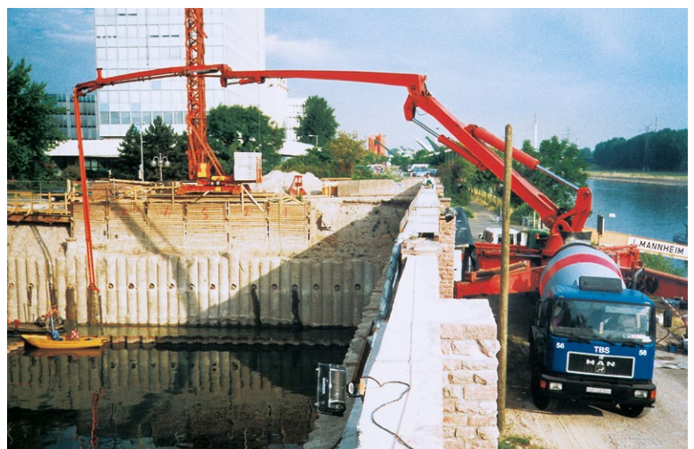
Rainwater overflow tank under construction in the city centre in 1997
